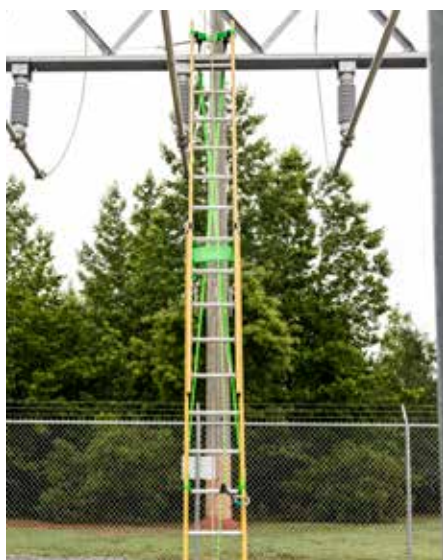
Front view of BLT attached to trussing.
