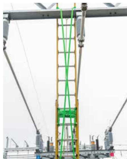
Rear view of BLT attached to trussing.
