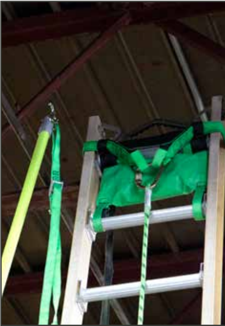
1. Once ladder is in place, use telopole to lift BLT straps over lattice.
