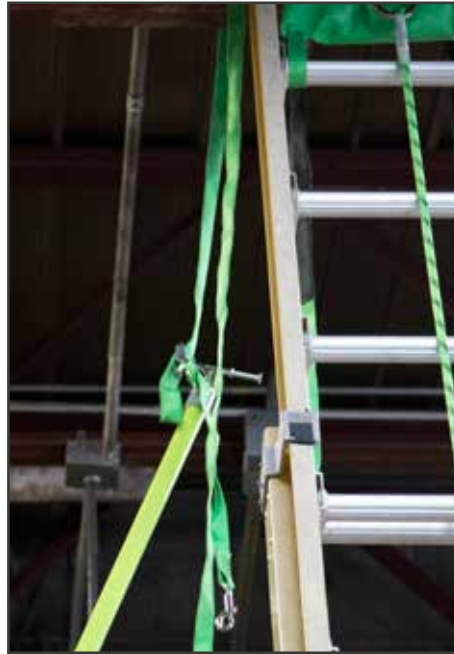
2. Pull straps down using telopole.
