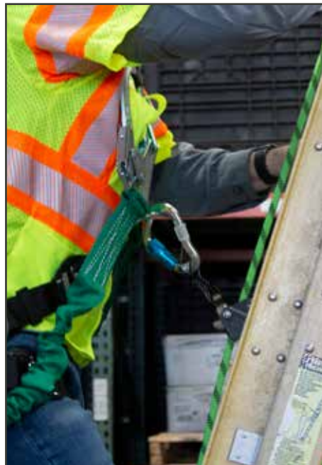
5. Attach carabiner of mobile fall arrester to sternal D-Ring on harness.
