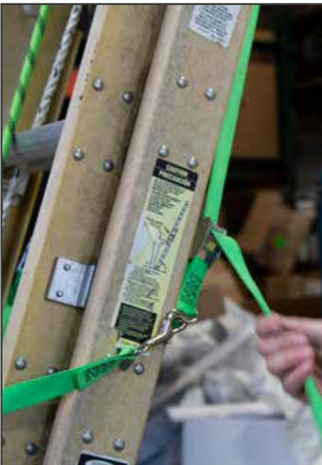
4. Attach straps to rails on ladder.
