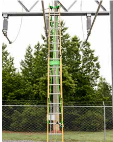
Front view of BLT attached to trussing.
