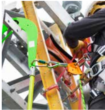
3. Attach MFA to lifeline, and the lifeline to sternal harness attachment and you are ready to climb 100% fall protected!
