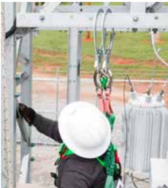
Big BuckSnaps™ attached to the Versa-Yard™ and attached over angle iron.
