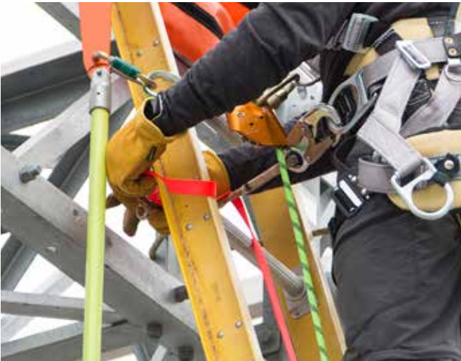
Installing upper stabilizer strap of Ladder Lock (model 355T) w/fall protection. Being used w/BuckHook™ Climbing System. See Pg. 23 for more info.
