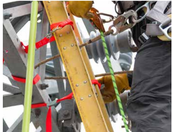
Ladder Lock (model 355T) used to secure top of ladder prior to working.
