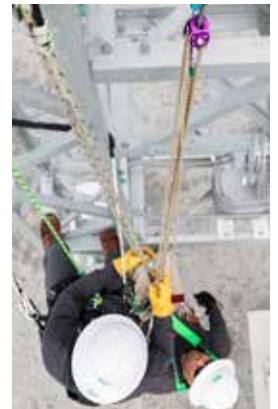
3. Rescue, lowering with the OX BLOCK™. See page 30 for OX BLOCK™ & accessories.
