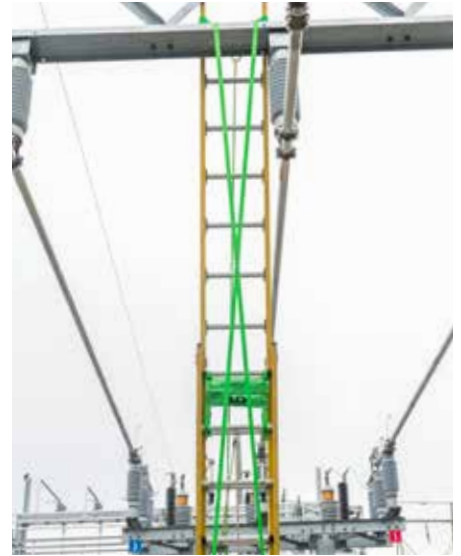
Rear view of BLT attached to trussing.
