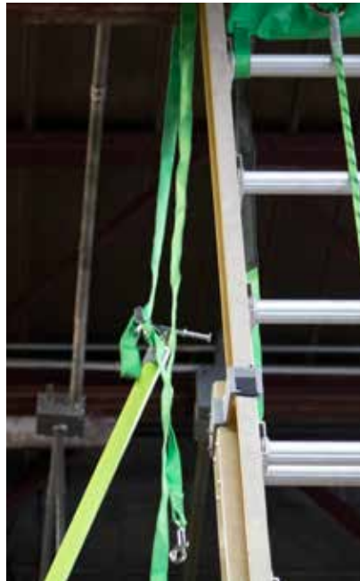
2. Pull straps down using telopole.
