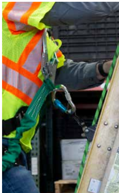
5. Attach carabiner of mobile fall arrester to sternal D-Ring on harness.
