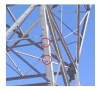
3. Standard, non-BuckBolts are not engineered to use as fall protection anchorages.
