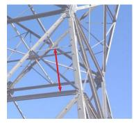
4. You can still fall more than 2 feet if rigged incorrectly using a work positioning lanyard on a vertical leg.
