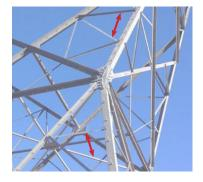
2. Many pieces of angle iron are not rated to use as fall protection anchorages.
