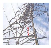
1. On certain structures, angle iron can be very far apart, making it difficult to reach. Often times, one must climb up to connect then climb back down to disconnect the other leg of the lanyard. This takes twice the amount of climbing which is time consuming, tiring, difficult to do, and can lead to preventable injuries. With BuckBolts, the user cuts their work in half.
