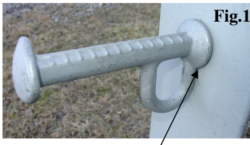
Mount Flange Flush to Support Structure
