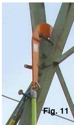
b. Insert rope into channel of Fall Arrester
